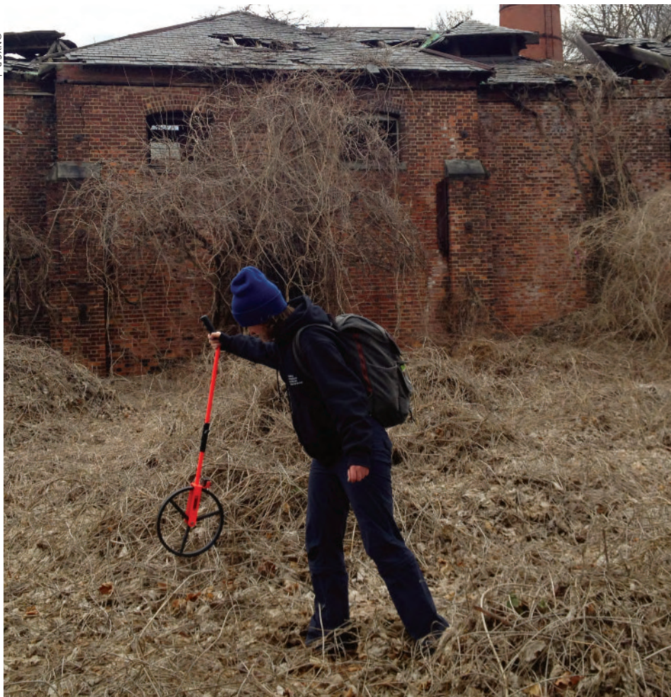
Kristen King Takes Measurements in Preparation for Restoration Work on North Brother Island
